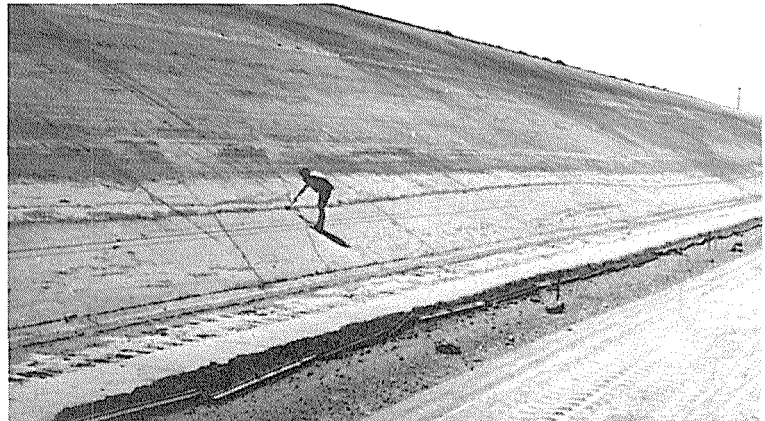
FIG. 3 Four filled cracks in the trimmed bank of the San Luis Canal. Clay layer (marked by hammer) is not offset by cracks.
