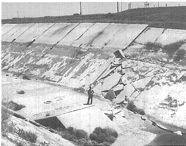
FIG. 3. Hydrocompaction damages to a test section of the State of California prototype canoe in the San Joaquin Valley.
