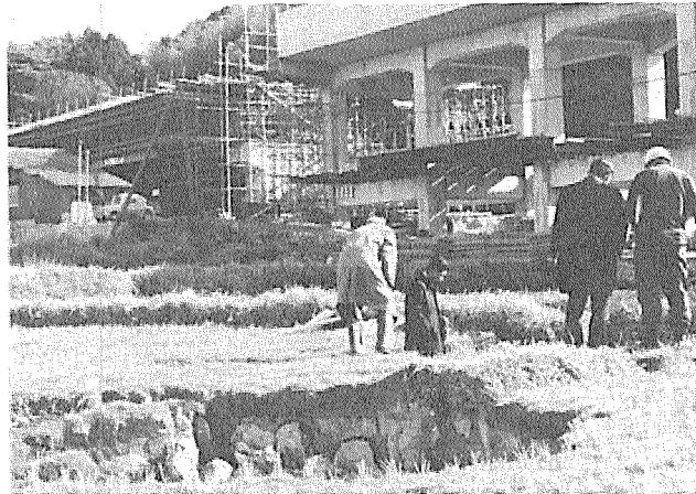
FIG. 3 Cave-ins due to ground water drainage.
