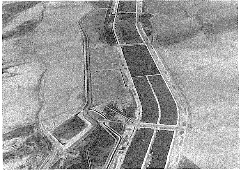
FIG. 5 Preconstruction flooding of one of the sections of San Luis Canal, California.
