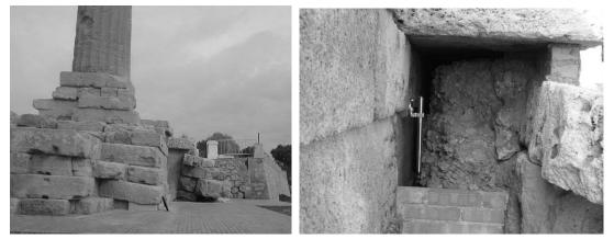
Fig. 5 Clinometer location in the base of the Doric column.
