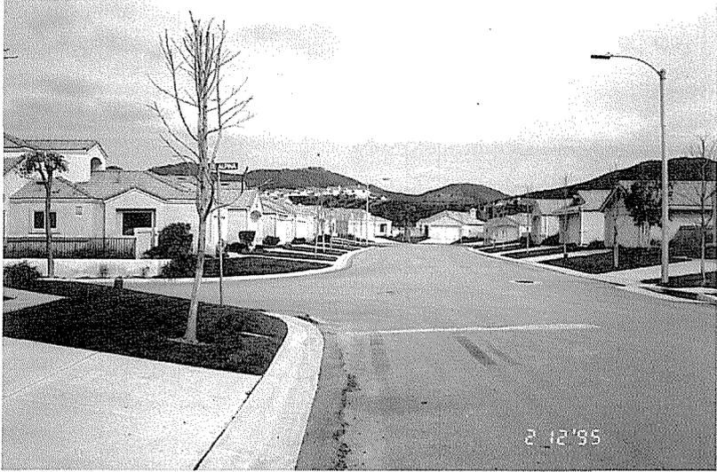
**Fig. 4** Unsold or abandoned "new homes" distressed by ground fissures and differential settlement. Disruption of street paving (foreground) is caused by subsurface soil hydrocollapse resulting in street tilting and 10 cm of surface compression. The concrete curbing, acting as a temporary rigid beam, is now cracked.
